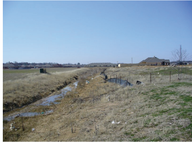
Figure 5. Field site #34, example of site designated as WQCM lowest priority quartile.
