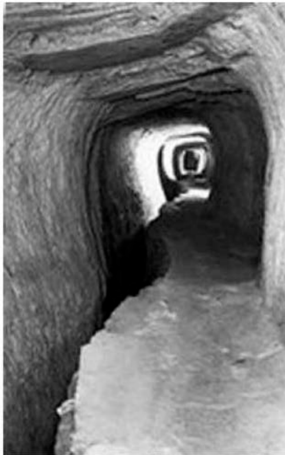
Figure 7. The aqueduct of ancient Samos [16].
