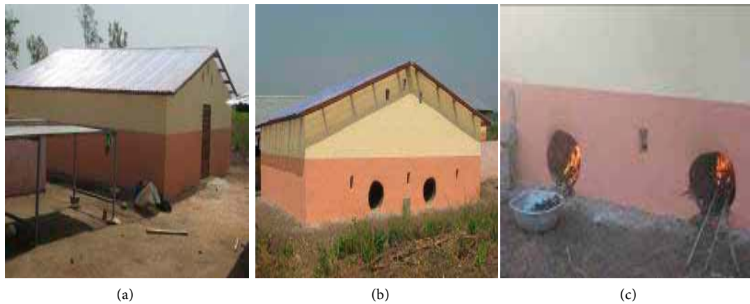
Figure 2. (a) Drying House; (b) Plastic Roof; (c) Heating Chamber.
