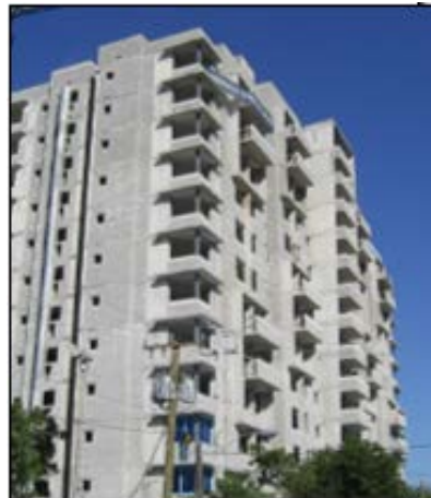
Figure 8. Photograph of building with reflective masonry insulation.
