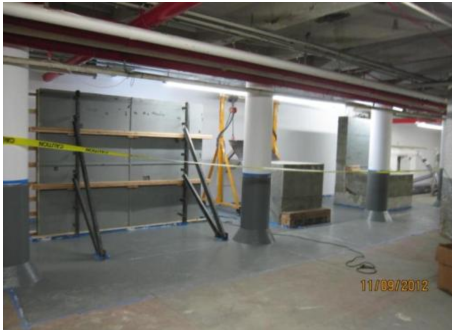
Figure 9. Appearance of the three fully constructed mock-ups.
