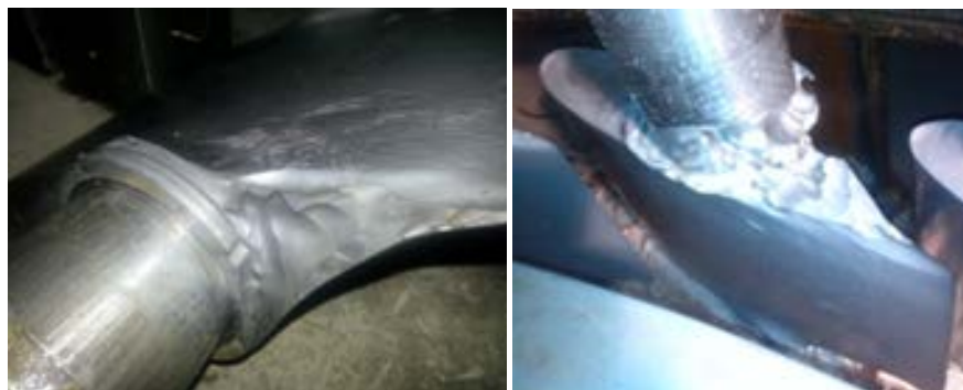
Figure 1. Erosion on turbine guide vanes.
