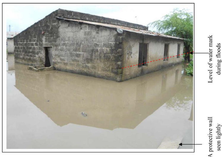
Figure 4. One of the respondent's houses surrounded by floodwater. Source: Photographed by T. Sakijege.
