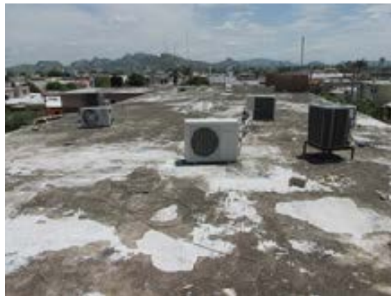
Figure 4. Roof of the main building with south view. Source: Own elaboration.
