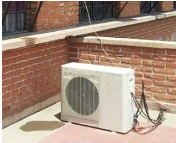
Figure 6. Mini-split type AC unit without lining. Source: Own elaboration.
