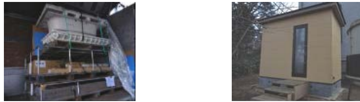
Figure 3. Packing of a bath-unit and a test house (1.4 m × 2.7 m) with a bath-unit.
