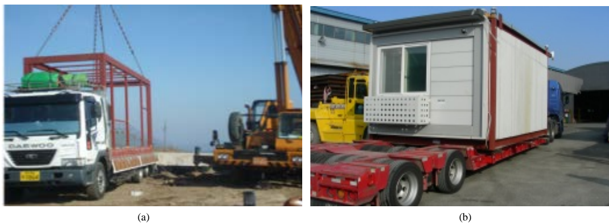
Figure 1. Unit modules' prefabrication percentage [6]. (a) 40% - 50%; (b) 80% - 90%.
