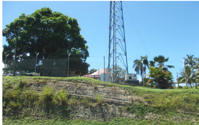
Figure 8. Location of the Suva GPS-station on a hill at an elevation of +73 m. The bedrock consists of gently dipping sedimentary rocks of questionable stability. The station has been classified as “non robust” and was deactivated in 2002.
