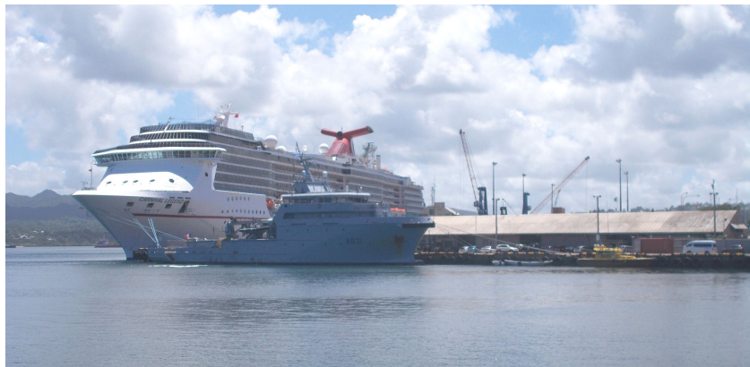
Figure 7. The tide-gauge station is located at the main wharf of Suva consisting of heavy construction resting on soft marine sediments. The load is bound to generate site-specific subsidence, seriously affecting the tide-gauge record.
