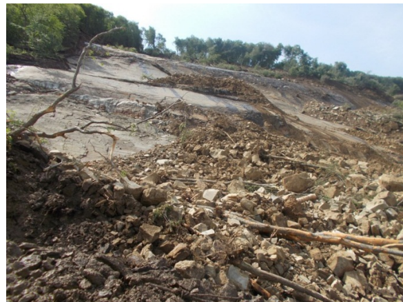
Figure 3. Sandstone blocks and fractured rocks remain on the slope.
