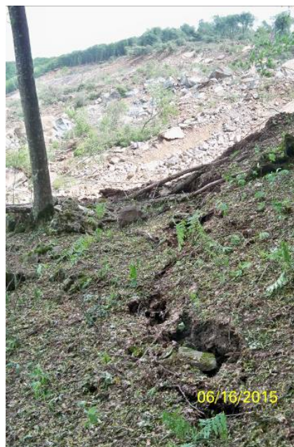
Figure 10. Fractures on Akhaladaba big landslide.
