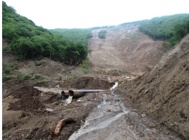
Figure 16. Destroyed Tskneti-Akhaldaba road.
