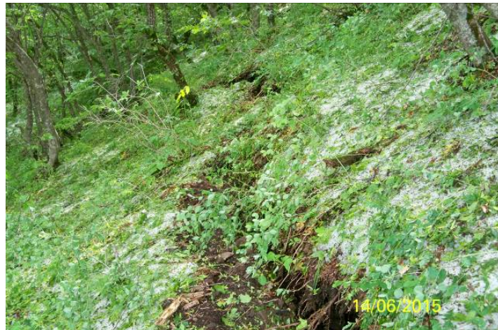
Figure 7. Fractures on Akhaldaba big landslide.
