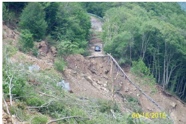
Figure 15. Destroyed Tskneti-Samadlo road.
