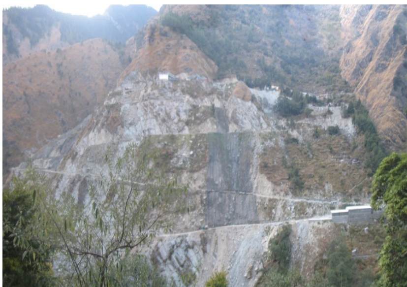
Figure 5. Debris deposits and mass wasting along the road access to the Gungaadit.
