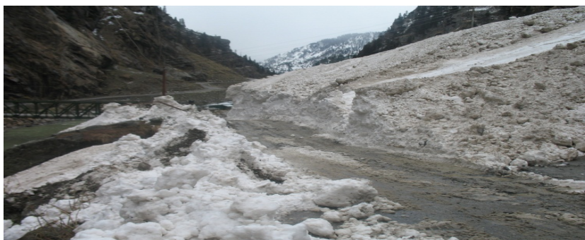
Figure 2. Avalanche at Dabrani Adit across the National Highway 108 (NH-108).
