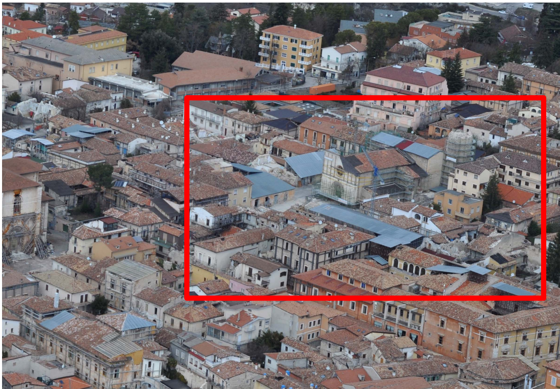
Figure 2. The church of S. Pietro a Coppito and the nearby buildings in March 2012.
