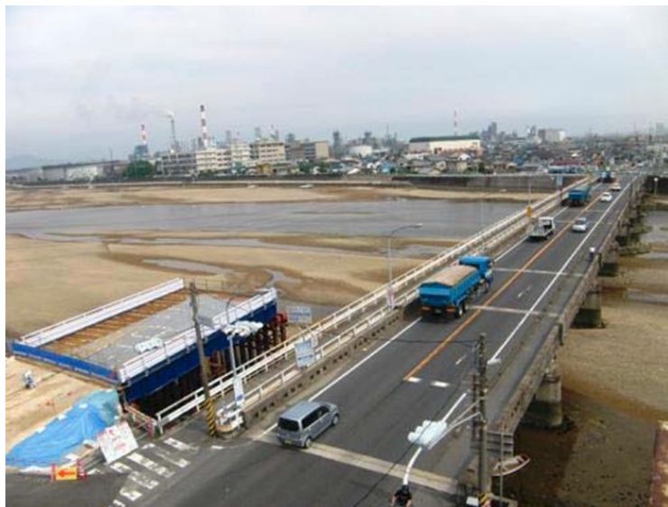
Figure 27. General view of the field test bridge (Sakae Bridge) when in service.
