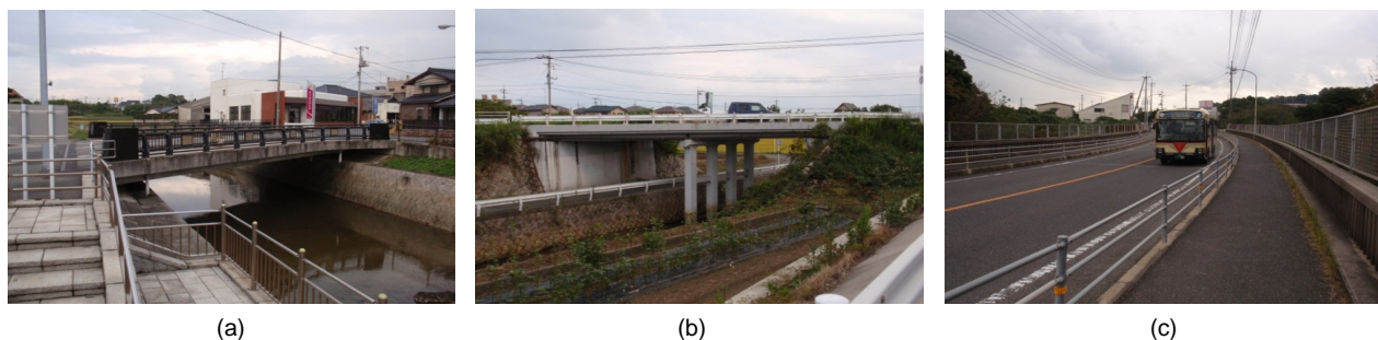
Figure 12. General views of Ube-city bus route bridges selected for long-term monitoring. (a) Shingondai Bridge (single-span bridge); (b) Shiratsuchi Daini Bridge (two-span); (c) Jase Bridge (five-span bridge).
