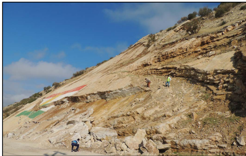
Figure 2. General view of Koya Landslide (the slid mass is removed).
