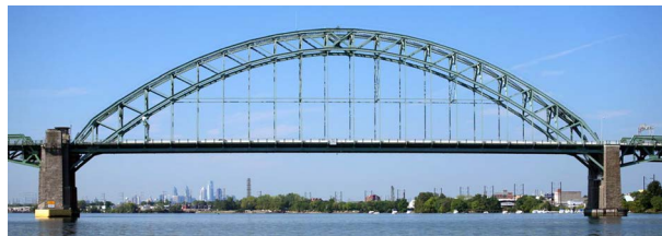
Figure 2. Steel tied-arch bridge photo.
