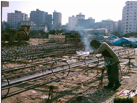
Figure 6. Fabrication of steel cage at site.
