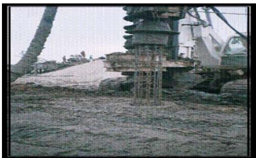
Figure 8. Reinforced steel cage inserted in concrete column by vibration.
