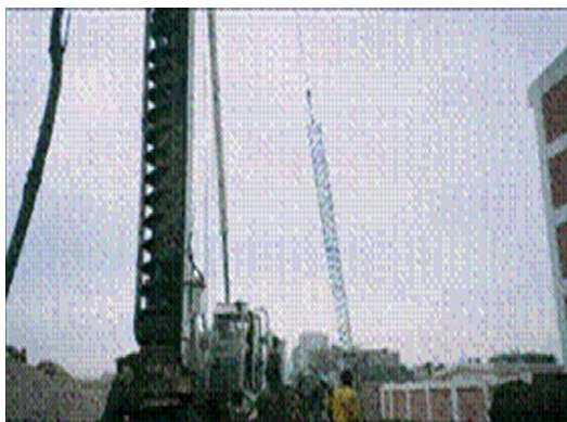
Figure 7. Drilling and concreting of pile by (CFA).
