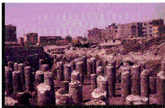
Figure 12. Site after excavation to requirement dept of raft foundation.
