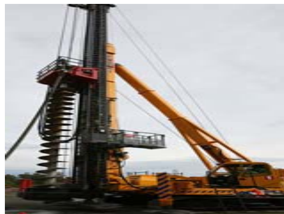
Figure 5. The machine used in execution of (CFA) piles.
