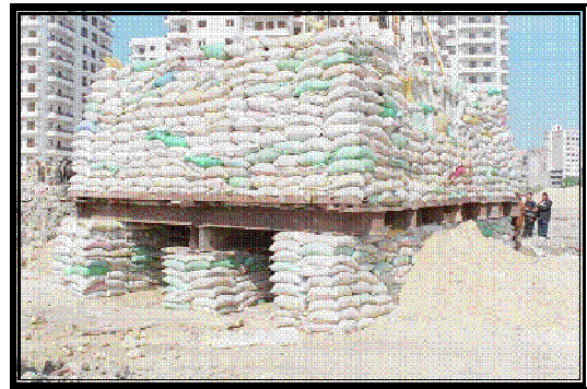
Figure 10. Knetledge method for pile test.
