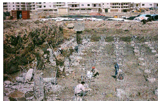
Figure 13. Remove of pile concrete head.
