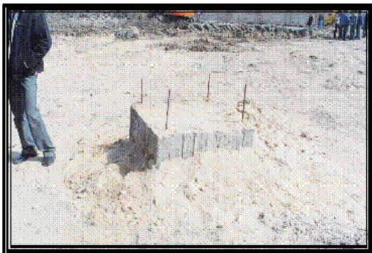
Figure 9. The pile cap of tested pile.
