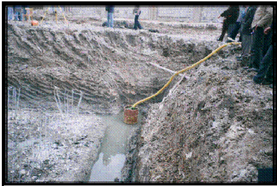
Figure 14. Surface dewatering of ground water for the site.
