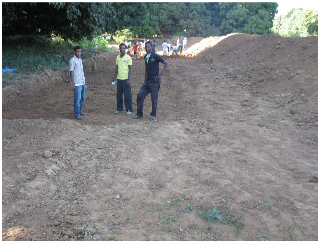
Figure 4. Students digging the pond.
