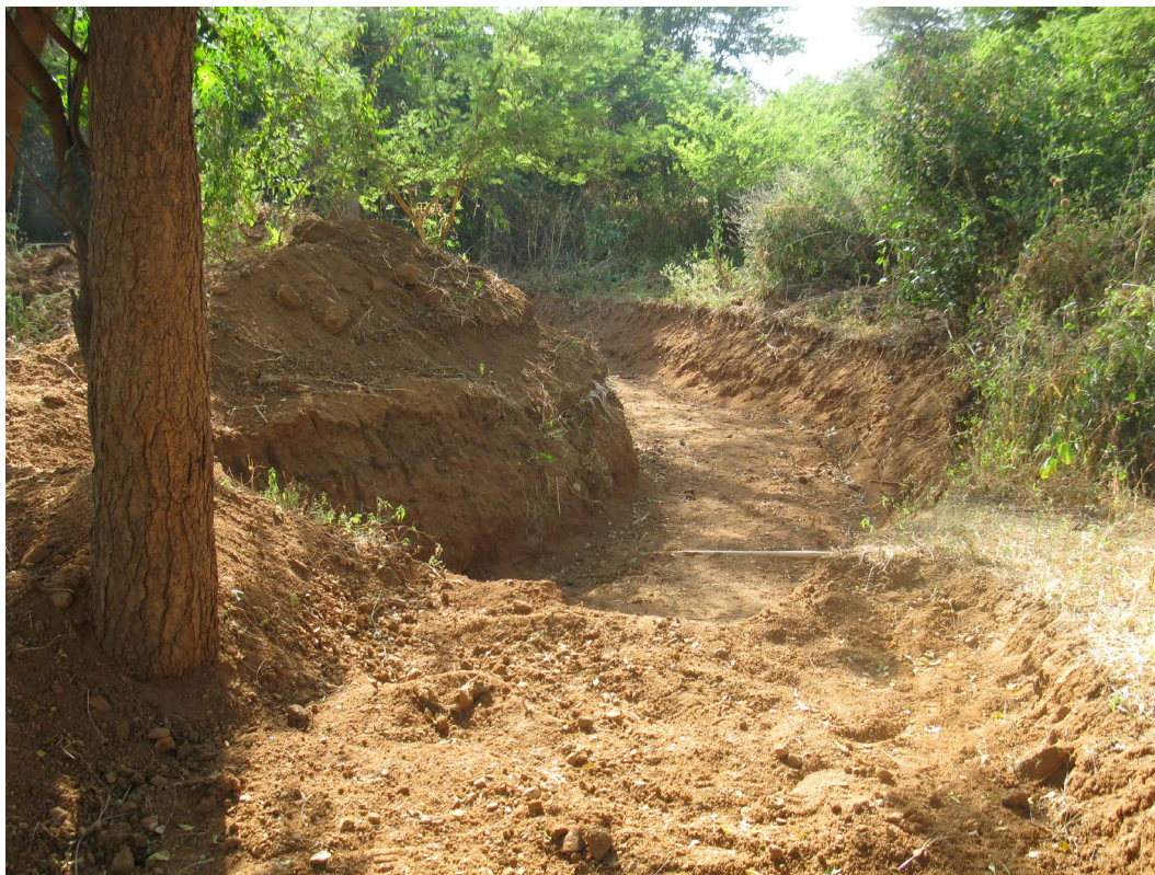
Figure 3. Waterway to intercept runoff.
