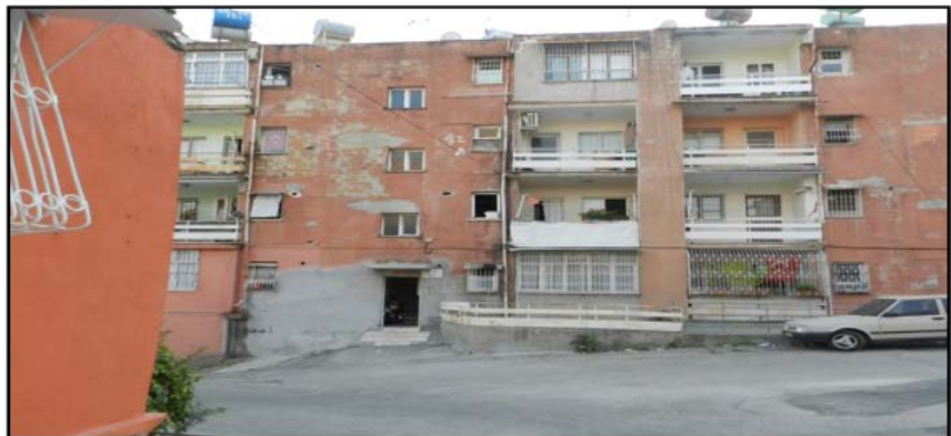
Photo 3. Present day four storey buildings in Belediye Evleri neighborhood.
