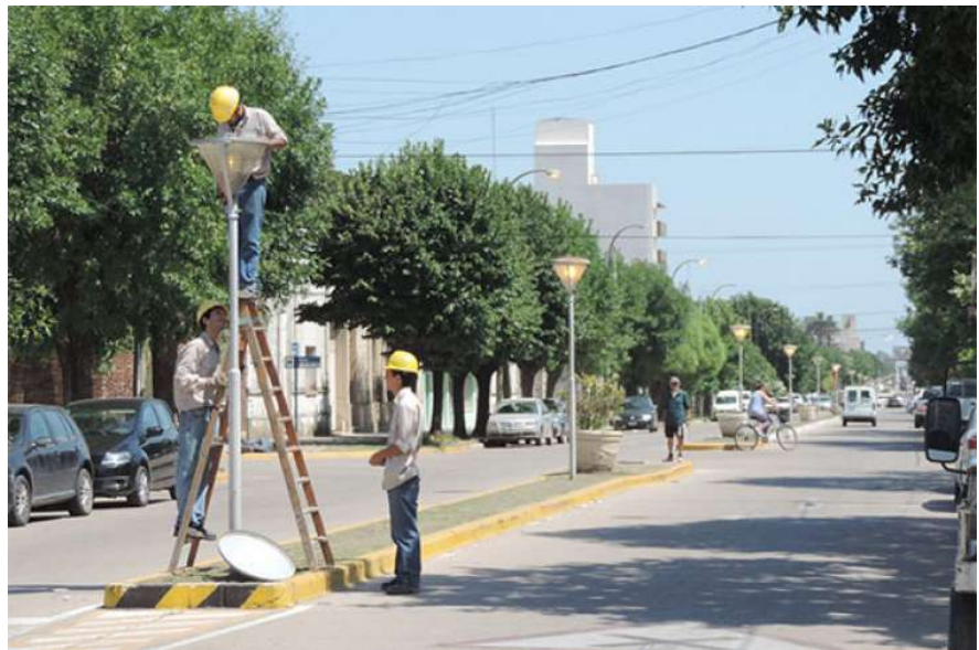
Photo 4. CEyS personnel repairing street lamps (Source: DiarioTiempo Digital , January 7, 2018) 20 .
