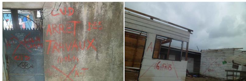
Plate 2. Buildings earmarked for demolition in Douala V local council. Tende, October 2017.
