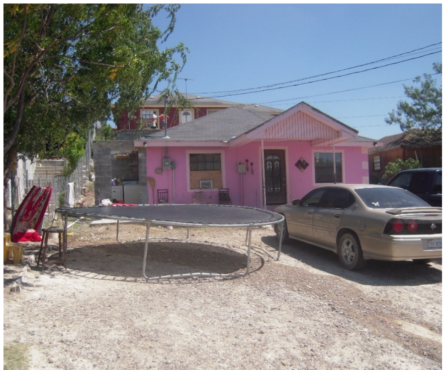
Figure A4. Shared lot with two self-built homes. Upper level is elderly parental home (red) and lower level daughter's family home (pink). Steps at side (invisible in photo) are steep and have hazardous unprotected drop on one side. (The two households plan on flipping their residence as the parents get older and struggle with mobility.) Author's photo (Ward).
