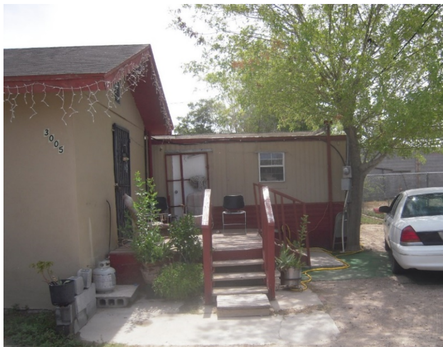
Figure A2. Hybrid dwelling structure comprising manufactured (trailer) home tied into a later self-built dwelling unit (on left). Author's photo (Ward).
