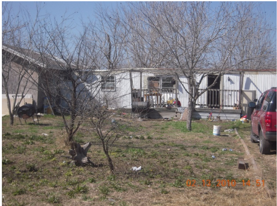
Figure A1. Dilapidated manufactured (trailer) home tied into a self-built (unfinished) dwelling unit (on left). Typical yard in winter. Author's photo (Ward).
