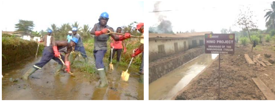
Plate 1. Labour intensive dredging project (HIMO) of stream channel in Kumba. Source: Fieldwork, January 2015.
