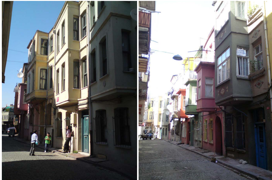
Figure 5. Row houses of Fener. Photo: S. Mijdem Vural.
