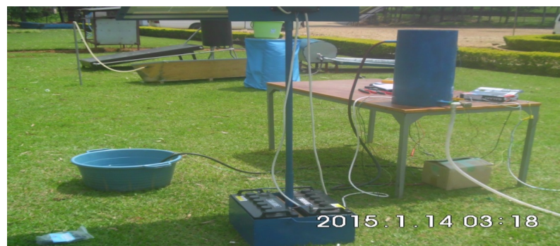
Figure 3. Test arrangement of automatic solar pumping system for irrigation.
