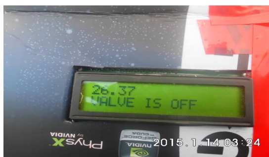
Figure 6. Valve is off.
