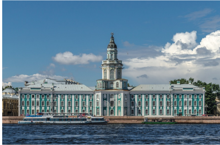
Figure 2. Original building of the imperial academy of science.
