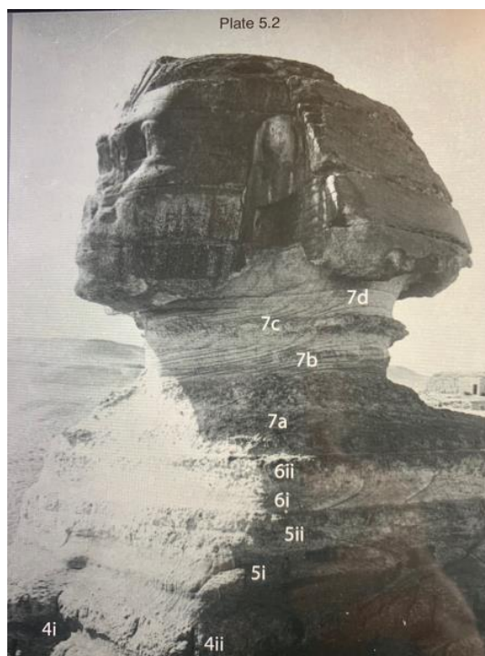
Figure 18. Gauri’s nomenclature labelling the individual substrata of the Upper and Middle Members (III and II) of the Mokattam Formation as they contribute to the head, neck, and body of the Great Sphinx. From Lehner (1991). The Archeology of an Image: The Great Sphinx of Giza . Zenodo. https://zenodo.org/record/1203621
