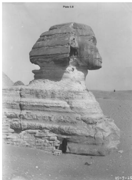
Figure 15. Pre-reconstruction photo from 1925 showing the frontal fissure vertically extending into the body of the Great Sphinx. From Lehner (1991) . The Archeology of an Image: The Great Sphinx of Giza . Zenodo. https://zenodo.org/record/1203621
