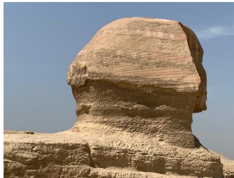
Figure 5. Converging Nemes headdress lines are still distinctly evident. Softer strata were filled in with concrete in 1926, during Émile Baraize excavation. The breakage scar at rear of head is clearly visible. Photo by R.S.N., June 2019.
