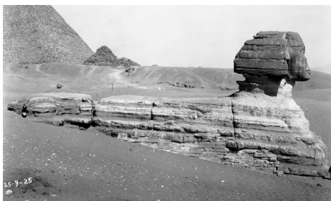
Figure 3. 1925 view of the Great Sphinx pre-restoration, before concrete repairs applied during Émile Baraize’s excavation. The Major Fissure at hips of the statue is still visible, in addition to the crack directly behind the head. The front fissure possibly was created during the same impact which caused the royal Nemes tail to break off.
