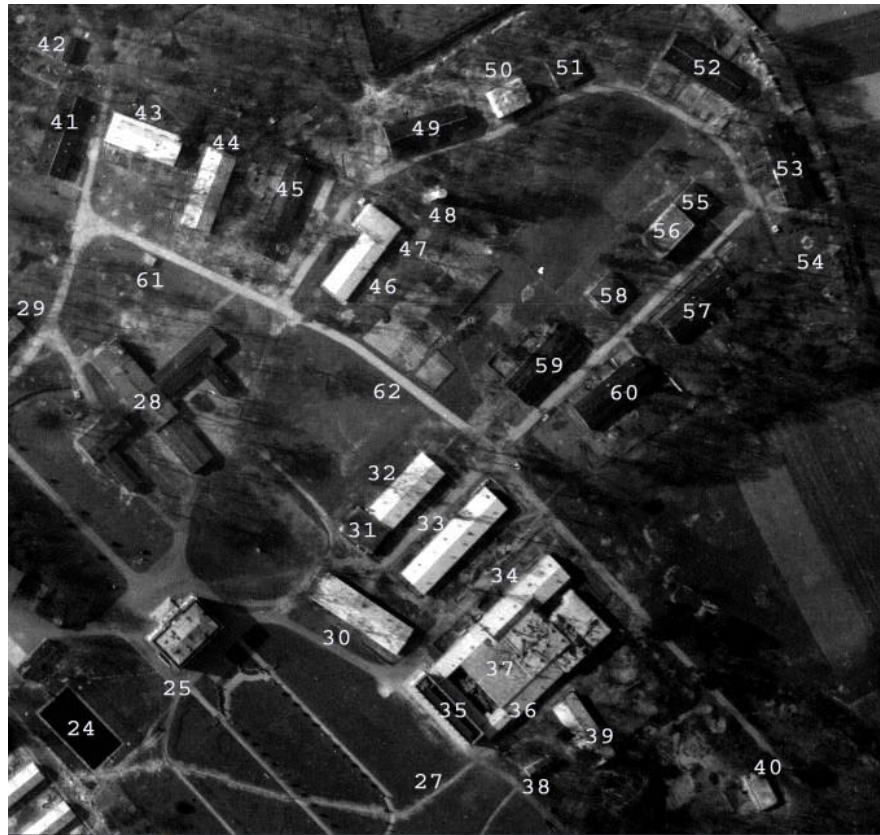
Figure 3. BDU organization—North part: (24) pool; (25) castle; (27) internal path; (28) administrative building; (29) - (30) barrack; (31) bunker; (32) (33) barrack; (34) barrack leaning to the Admiral bunker, (35) orangery, (36) barrack leaning to the Admiral bunker, (37) Admiral bunker, (38) (39) barrack; (40) bunker, (41) - (46) barrack; (47) bunker; (48) water tower; (49) barrack; (50) bunker; (51) - (53) barrack; (54) possible Flak position; (55) barrack leaning to the bunker (56); (56) bunker; (57) - (61) barrack, (62) internal path.
