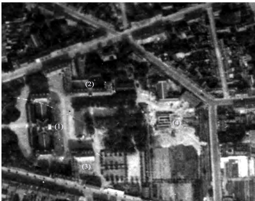
Figure 8. UCO campus—(1) university Palace; (2)-(3) university buildings; (4) excavation and R 608 C1522-0421_1944_US7GP2926_2021, n°2012, 1/9980, Argentique, 14/08/1944.
