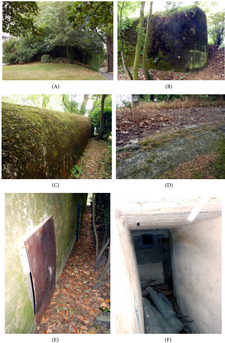
Figure 16. Bessonneau bunker—(A) exterior appearance; (B) and (C) external concrete structure; (D) coverage; (E) metallic plates blocking the entrances; (F) entrance corridor, on the top, louver of the close combat room, on the right rusty heavy metallic door 434PO1, on the floor, metallic conduits.
