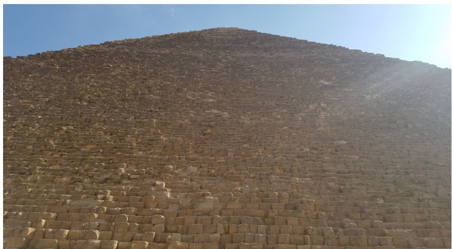
Figure 2. View of the west wall of Khufu's pyramid on a winter afternoon with the sun rays approximately parallel to the east and west base. The concavity is produced by an indentation which displaces the core from the original cased perimeter by a maximum of 0.92 m at the side centers, 220rc from the corners. Photo taken by the author in February 2017.
