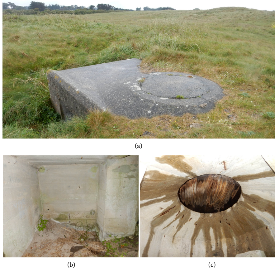
Figure 17. 3 rd tobruck (a) entrance and aperture of the combat room covered by a concrete layer; (b) entrance room partially invaded by sand and debris; (c) combat room, on the right step protruding from the wall, on the upper side aperture closed by wooden boards.
