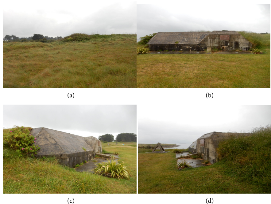
Figure 14. V2d at Corn ar Gazel beach (a) connection trench; (b) front vision; (c) side vision; (d) side vision, on the left concrete tetrahedron.
