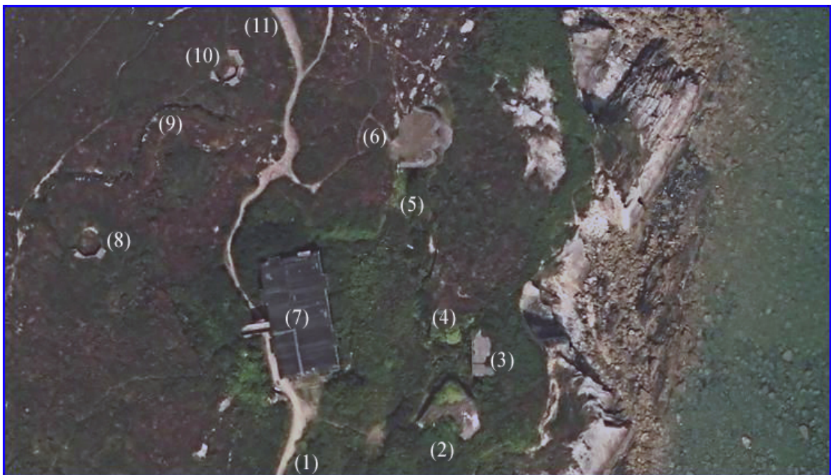
Figure 3. Petit Gouin pointe (1) access pathway, (2) 1 st R670 , (3) 1 st barrack, (4) 2 nd barrack, (5) concrete platform, (6) 2 nd R670 , (7) French crenelated guardhouse, (8) 1 st 2cm Flak gun 30 emplacement, (9) connection trench (10) 2 nd Flak gun 30 emplacement, (11) pathway to the Grand Gouin pointe [GeoPortail].
