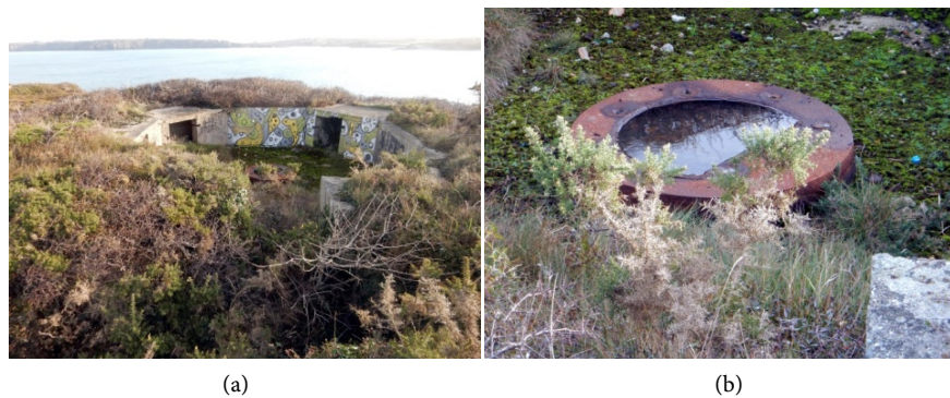
Figure 10. 1 st 2 cm Flak gun 30 emplacement (a) entrance and ammunition stores; (b) ground metallic support for the gun.
