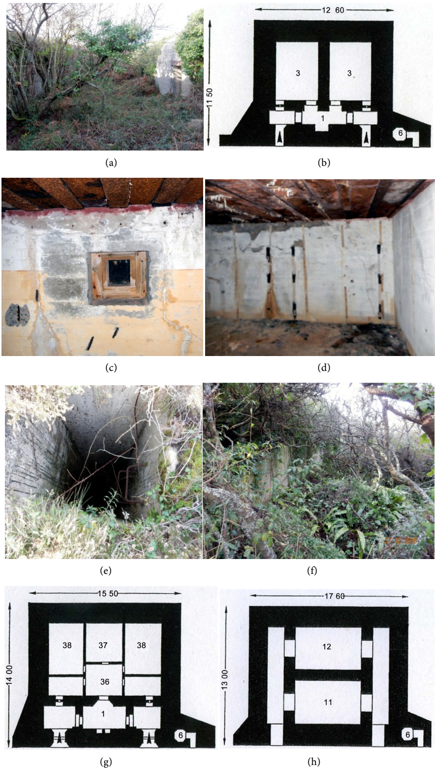
Figure 20. Facing H622 and H638 (a) on the left H638 on the right H622; (b) H622 plan. 1 gas lock, 3 crew room, 6 observation post (Rudi, 1998); (c) H622 entrance; (c) H622 crew room (d) crew room, on the wall cot support joints; (e) H622 escape conduit; (f) H638 covered by the vegetation; (g) H638 plan. 1 gas lock, 6 observation post, 36 admission room, 37 treatment room, 38 sickroom/ward (Rudi, 1998); (h) H641 plan. 6 observation post, 11 shells room, 12 cartridge room.
