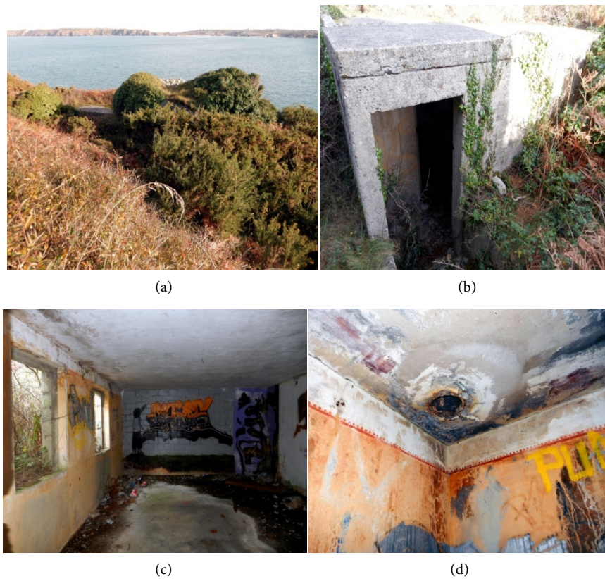
Figure 5. 1 st barrack (a) coverage, on the top Trez-Rouz beach “British Death”; (b) entrance; (c) lodging room; (d) chimney hole probably for Festungshofen (fortress oven) WT80.
