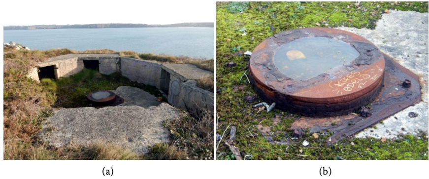
Figure 11. 2 nd 2cm Flak gun 30 emplacement (a) entrance and ammunition stores; (b) ground metallic support for the gun.
