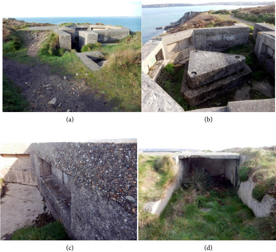
Figure 12. 150 cm search light emplacement (a) labyrinth entrance, on the left electric generator garage, on the right rectangular, concrete emplacement (b) interior with triangular concrete base with three recesses; (c) side niche; (d) electric generator garage.
