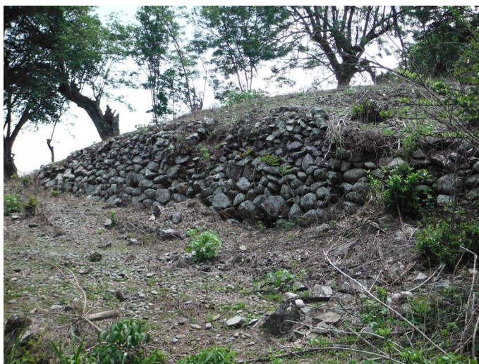
Figure 4. One of several rock retention walls or muros at the Hacienda La Moraga archaeological site, Rio Medio Cauca, Colombia. During Colonial gold mining, the rocks were removed from the streams and stacked so as to more easily access and process the fine-grained gold-bearing sediments. Similar muros can be seen in the small-scale gold mining area of Tadó, Dept. Chocó, Colombia (Restrepo Uribe, 2014; Silva Herrera, 2010).
