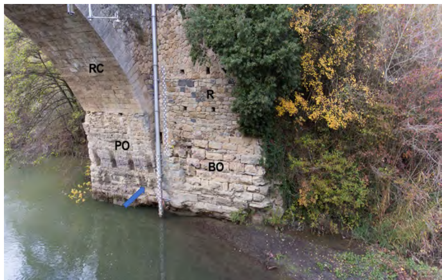
Figure 9. The photo shows, on the left bank of the Ofanto River, the reconstructed arch 1 (RC), the original structures of the pier (PO), from which the sample PO 11 of mortar highlighted by the arrow was collected, and, on the right, the base of the buttress (BO). The middle upper part of the buttress is restored (R) mainly with squared ash-lars of ACP Sandstones and some pebbles of dark gray siliceous limestone. The vertical tube is part of the hydrometric device.
