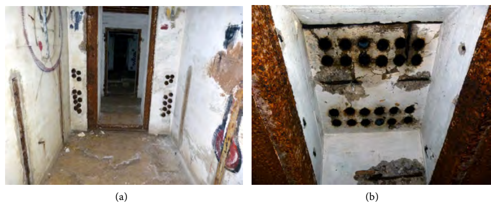
Figure 12. L 485 : (a) gas lock and antenna room; (b) antenna room ceiling.
