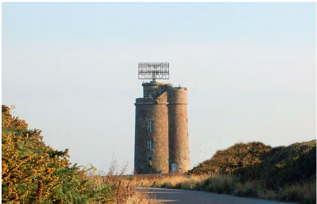
A1: reconstruction— FuMO 2 on top of the headlight for air and sea surveillance.
