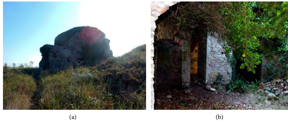
Figure 4. Stone and brick construction (3): (a) lower wing; (b) construction interior.
