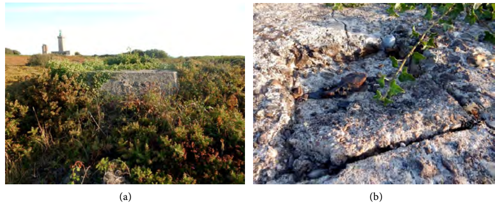
Figure 14. VF229: (a) support for Würzburg Riese ; (b) imprint of the radar connection.
