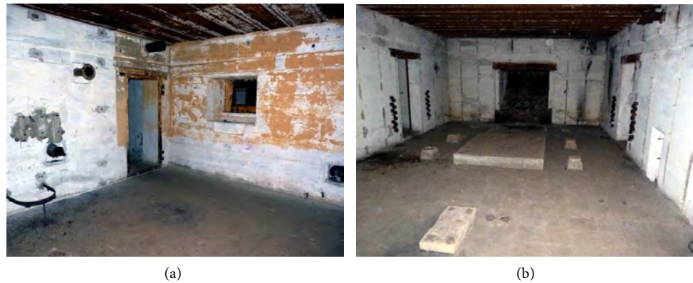
Figure 11. L 485 : (a) internal room, on the right wall defence loophole on the left wall metallic support of unknown purpose; (b) compensator room.
