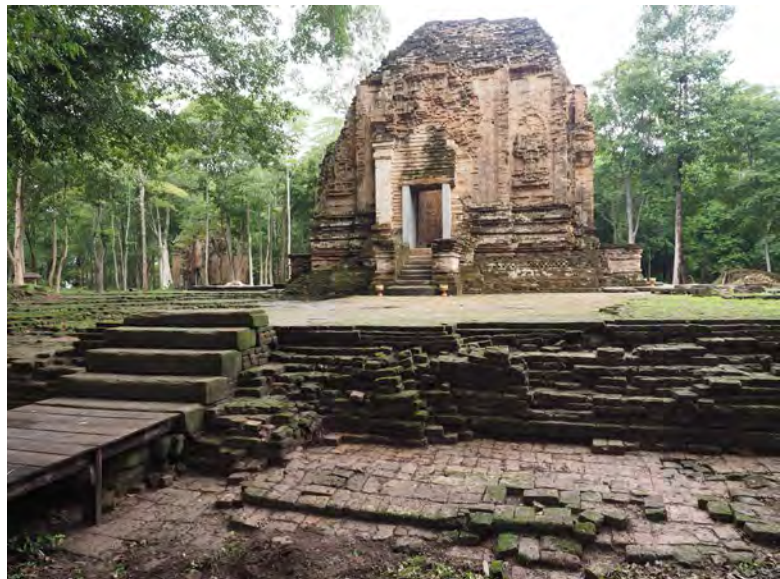
Figure 5. Central shrine (N1) standing on the central terrace of Prasat Sambor (view from north).
