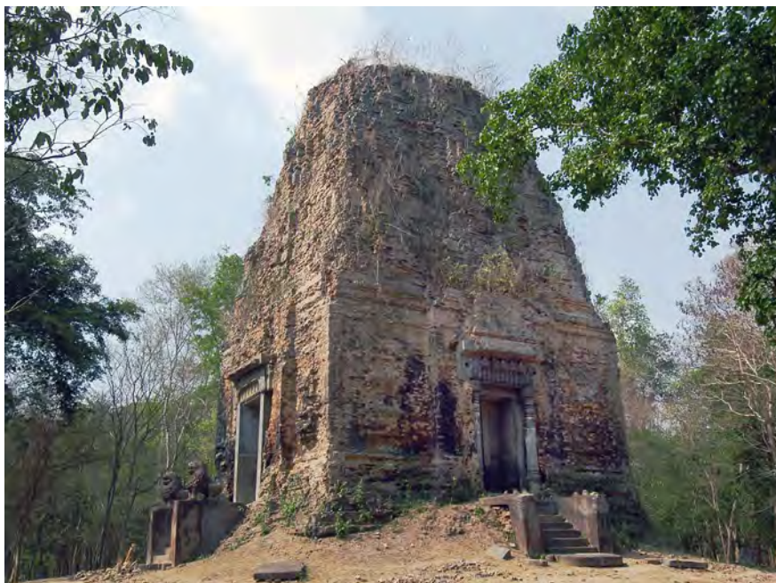
Figure 16. Central shrine (C1) of Prasat Tao (view from northeast); front door is opened and accessible to the chamber but other three sides are only decorated with false doors and steps.
