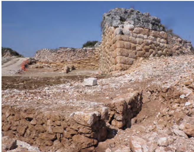
Figure 16. Temporary masonry foundations, adjacent to the edge of the tower.
