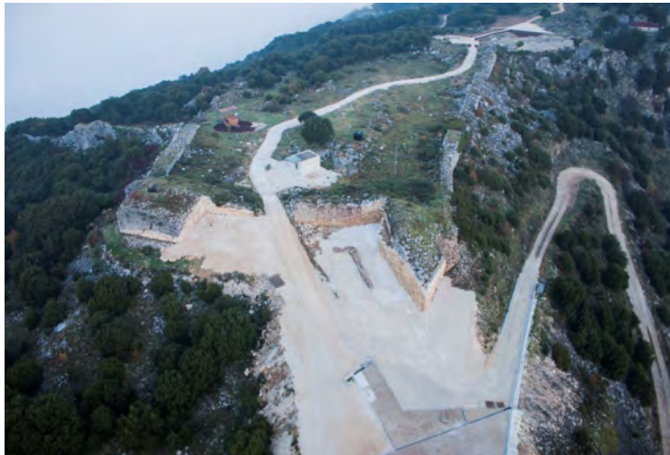
Figure 3. Aerial view of the eastern projection of the fortification.
