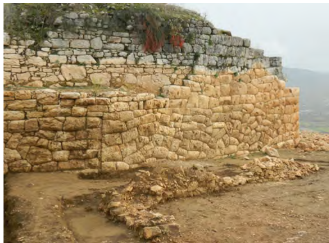
Figure 17. Temporary masonry foundations, adjacent to the edge of the tower.
