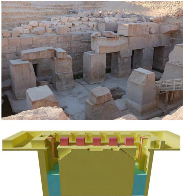
Figure 17. Top: Osireion , approximate south view looking north. Bottom: Graphic simulation of a vertical axial view of the Osireion as seen from the southeast looking northwest. This view gives a sense of the depth of the temple foundation including the observed (east) and predicted (west) horizontal thrust beams anchoring the temple walls to the island, and visualizes the stairs leading from the moat onto the island platform with its two quadrangular depressions possibly representing the two šbtjw, w3j / The Far and ‘3 / The Great (see Discussion ). The northwest row of granite pillars is highlighted in coral color and the sandstone pilasters/piers (outlined in coral) adjacent to these complete an apparent set of seven total pillars. Photo by R.M.S., June 2019; graphic design courtesy of Keith Hamilton; modified with permission.
