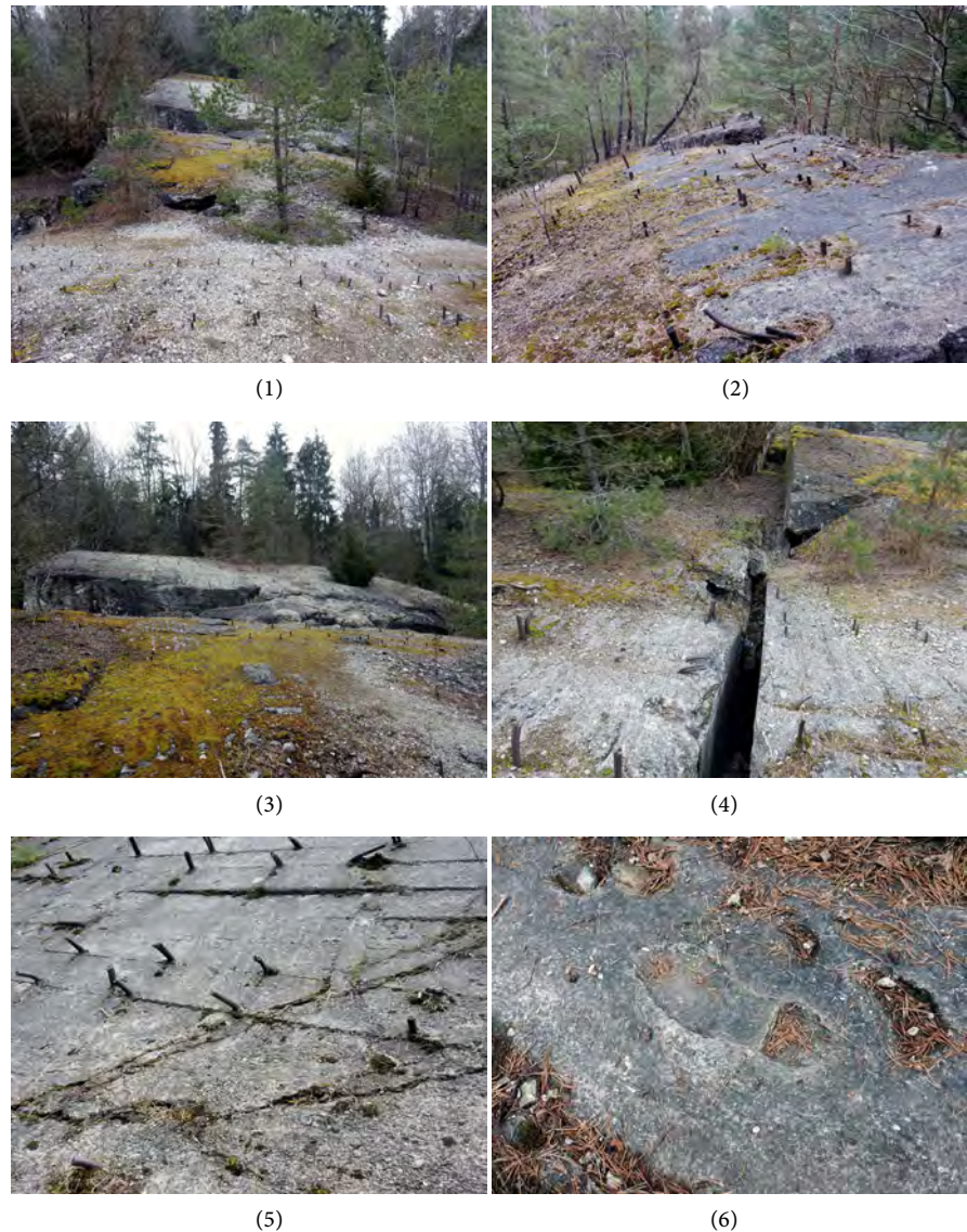
Figure 5. Weingut I —(1) 3 rd arch fractured coverage with aligned armour iron extremities; (2) 4 th arch fractured coverage with aligned armour iron extremities; (3) 5 th arch fractured coverage; (4) 30 cm gap between the 4 th and 5 th arch; (5) 6 th arch coverage with traces of the formwork elements and aligned armour iron extremities; (6) worker's shoe prints on the 6 th arch concrete.
