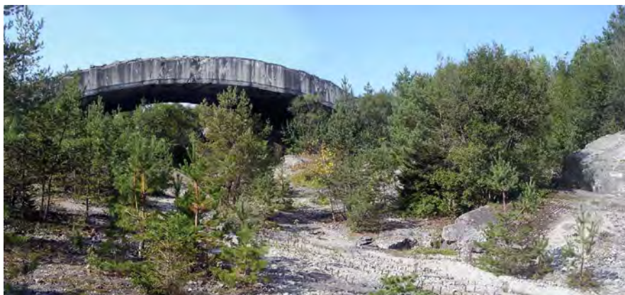
Figure 7. Weingut I—7 th arch, front side overview from the 5 th and 6 th arches.
