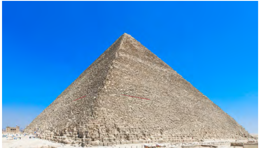
Figure 3. The 35 th course is marked in red on the north and west sides of the Great Pyramid. Photograph by Adobe Photostock, license # 102571012; modified.
