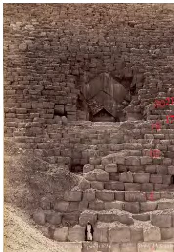
Figure 5. Main entrance to the Great Pyramid on its north wall. Shown in red are the course numbers and the tops of courses 17 and 21 are marked in red for orientation and to point to the thicker courses #18 and #22 immediately above. The thicker courses are immediately above in each case. Only #21 appears to mark a ceiling specifically the bottom notch of the lower pair of chevrons arching over the entrée. Note that this photo shows the Great Pyramid in its current state without the casing stones. Photo courtesy of Boston Public Library: “ The Entrance to Great Pyramid ” created by William Vaughn Tupper ( https://www.flickr.com/photos/boston_public_library/2469130012 ); modified. Creative Commons License.
