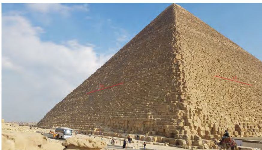
Figure 1. Southwest corner of the Great Pyramid showing the position of the 35 th course which runs immediately above the Queen Chamber's roof inside. The corner edge is one of four where Petrie made his measurement of course thickness up the 203 currently surviving course levels. Photograph taken by the author in February 2017; modified.
