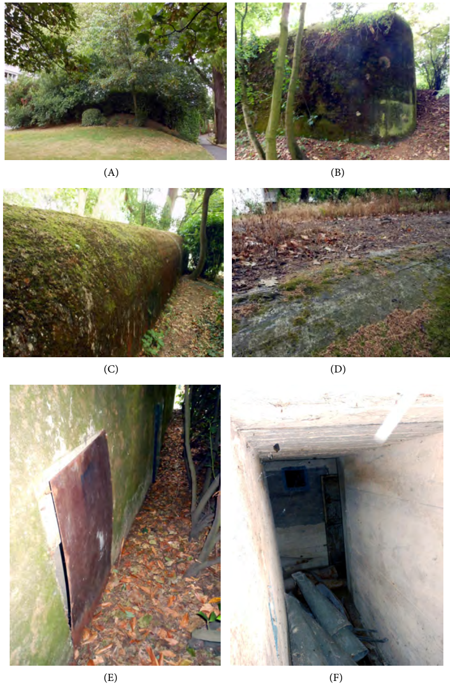
Figure 16. Bessonneau bunker—(A) exterior appearance; (B) and (C) external concrete structure; (D) coverage; (E) metallic plates blocking the entrances; (F) entrance corridor, on the top, louver of the close combat room, on the right rusty heavy metallic door 434PO1, on the floor, metallic conduits.
