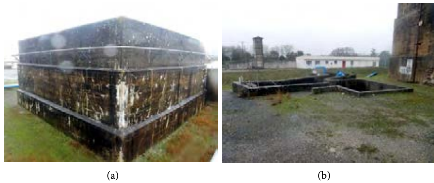
Figure 16. Bouchemaine oil terminal—(a) six sides wall; (b) after war manifold.
