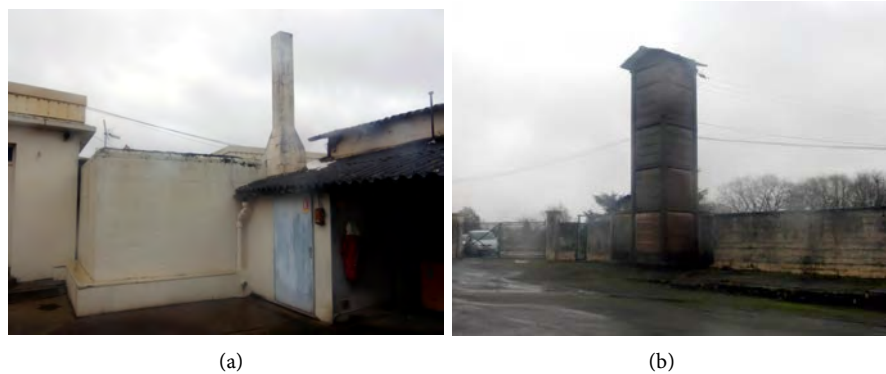
Figure 11. Bouchemaine oil terminal—(a) small German bunker h at the entrance; (b) after war electrical distribution cabin.
