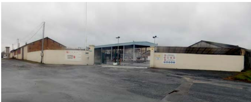
Figure 18. Bouchemaine oil terminal—present main entrance.
