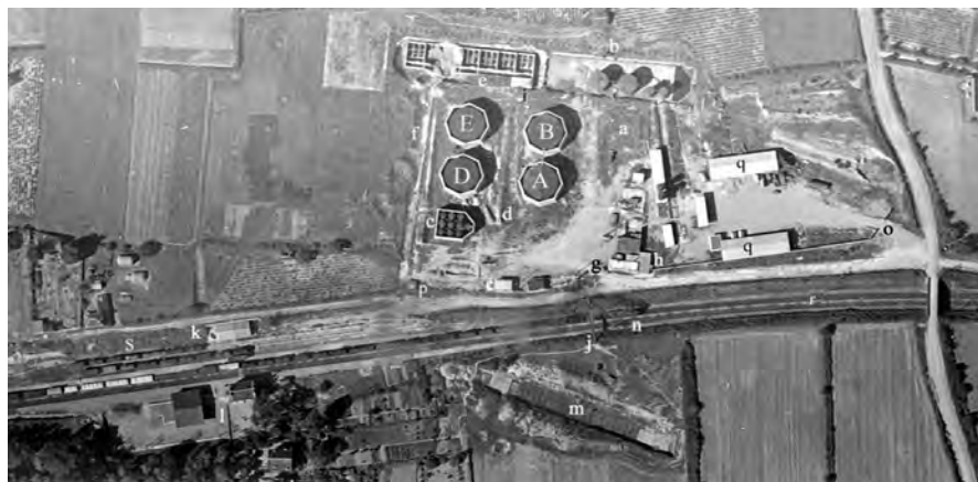
Figure 10. Bouchemaine oil terminal—a: 1st area; b: 2nd area; c: six side wall with tanks 1 to 10; A, B, D, E labelled octagonal walls and corresponding oil tanks; d: possible disappeared structure; e: damaged building; f: protected passage to the building e or anti-tank trench; g: terminal main entrance/exit; h: bunker; i: bunker; j: pipeline metal bridge; k: Bouchemaine freight station; l: Bouchemaine passenger station; m: excavation; n: train; o: entrance/exit p: minor construction; q: hangar; r: SNCF railway line, s: railway depot. (Mission identification: C93PHQ8041_1948_CDP3032_0010, cliché n° 10, scale: 1/5034, cliché type: Argentique, Date de prise de vue: 17/09/1948).
