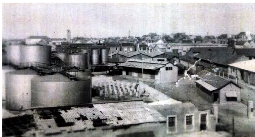
Figure 1. Talards oil terminal—pre-war image, on the left oil tanks, on the right entrance gate, on the foreground left the still existing square tower of the Civic Centre of the Louis Martin Avenue in front of the Commerce Chamber (Pottier, 2013; Archive Saint-Malo, 1940).
