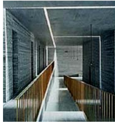
Figure 14. Fissure-light in the ceiling.
