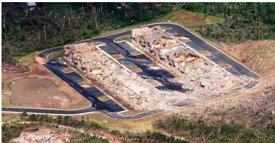
Figure 2. A tornado completely leveled an apartment complex in Tuscaloosa, Ala. (April 28, 2011). New York Times. http://www.nytimes.com/2011/04/29/us/29storm.html?_r=0
