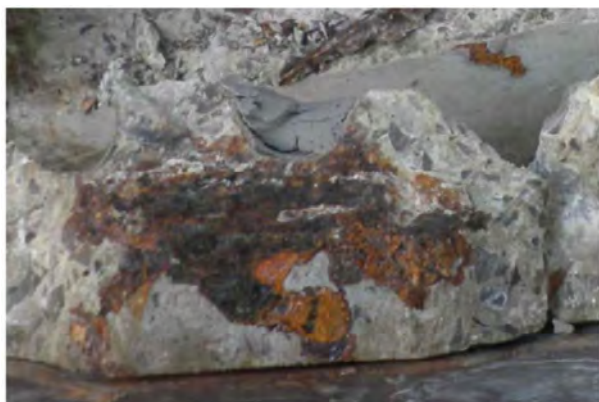
Figure 6. Staining and corrosion damage due to invasive attack of chloride.
