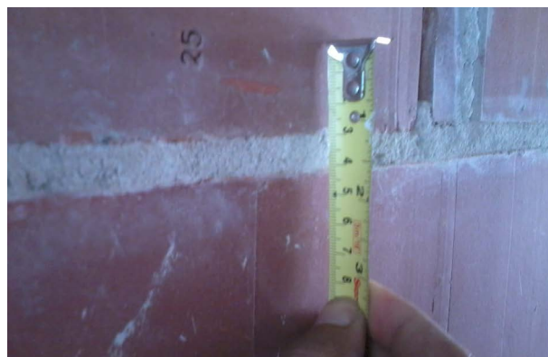
Figure 2. Joints within specifications.
