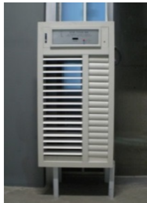
Figure 8. Complete view of double-blade air supply damper.
