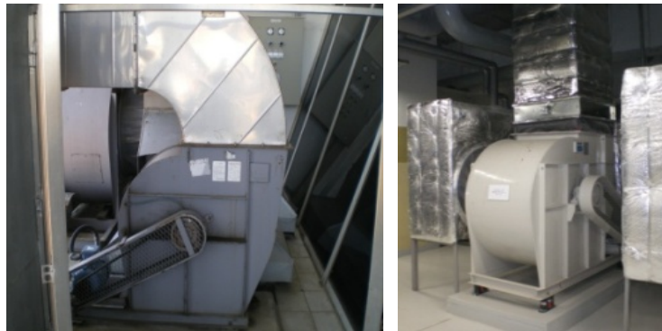
Figure 2. Air supply blower.
